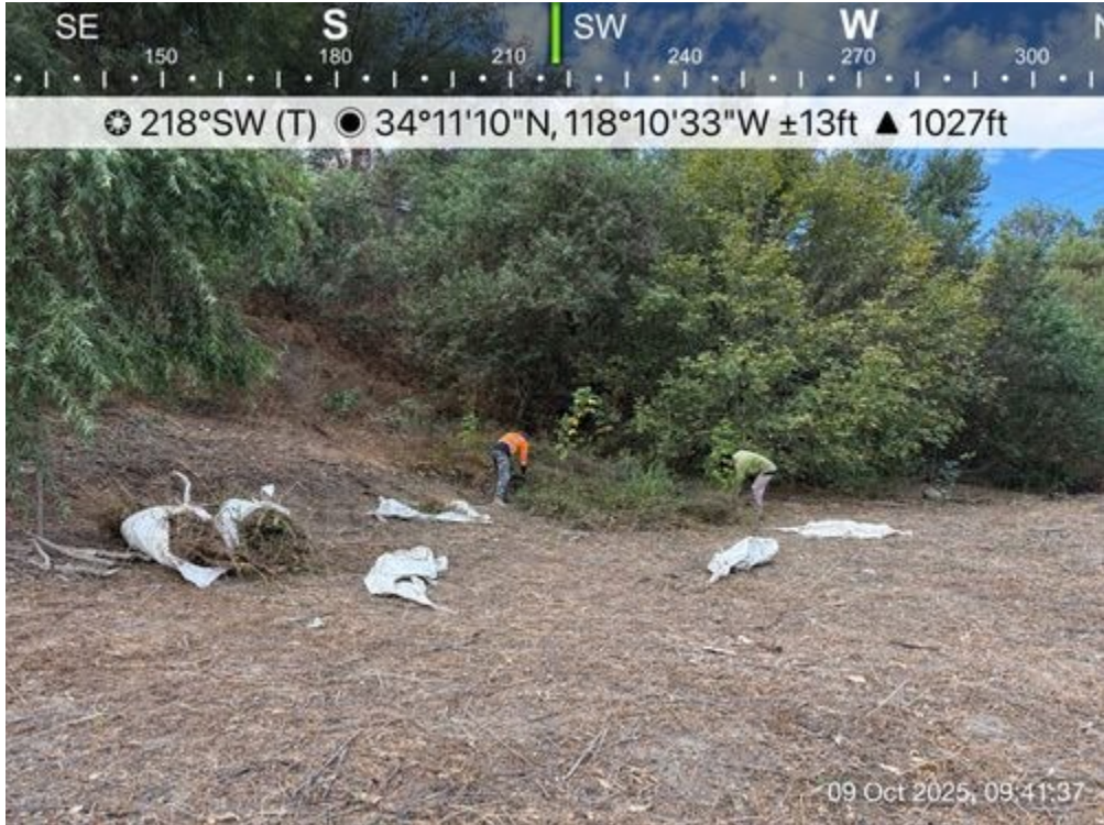
Vegetation Removal during facingSW.JPG -118.17599722222222 34.18613611111111
