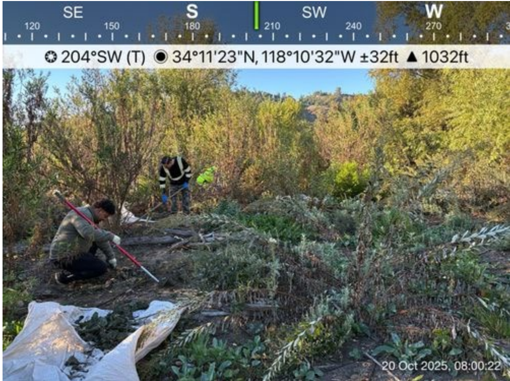
Vegetation Removal during facingS.JPG -118.17581666666668 34.18972777777776
